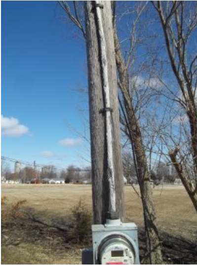
Sheathing on the wire coming out of the service meter to the overhead triplex cable is deteriorated and frayed
