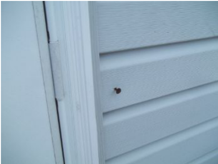
nails need removed
