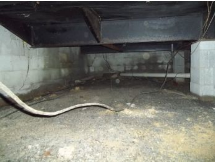
No piers at the end of steel frame
