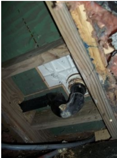
Shower drain appears to have a leak
