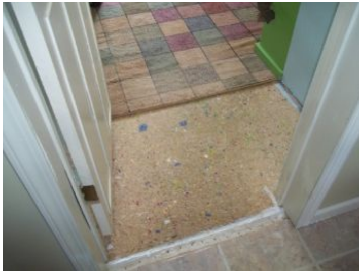
No floor covering in center bedroom
