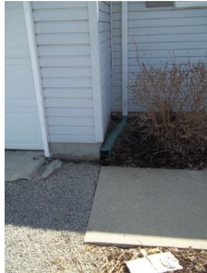
Downspouts discharging to close to the foundation
