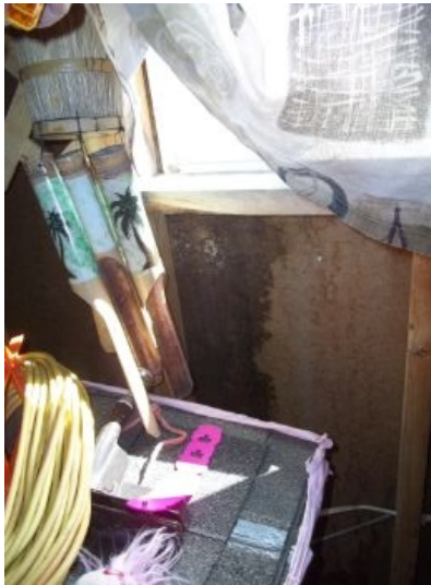
Rear garage window leaking, sub sheeting was wet under the window
