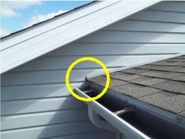
Roofer should have installed a kick-outs so water does not run behind the siding
