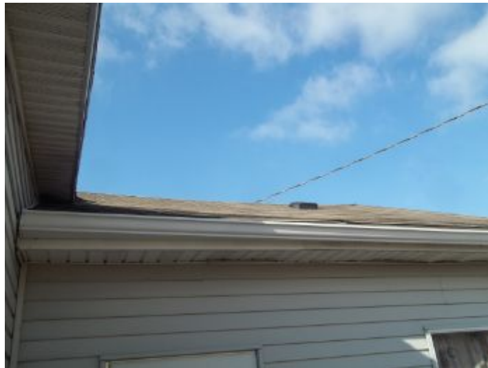
Garage roof sagging
