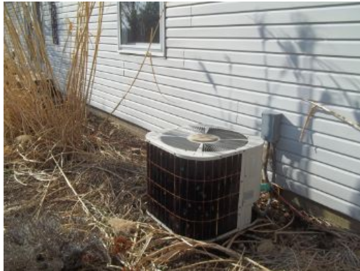
Data missing from AC unit, appears to be original equipment
