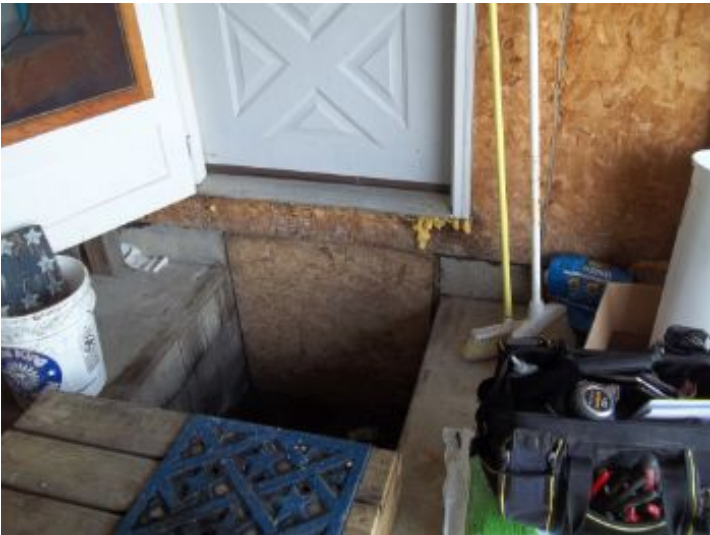
Crawlspace access in garage under step
