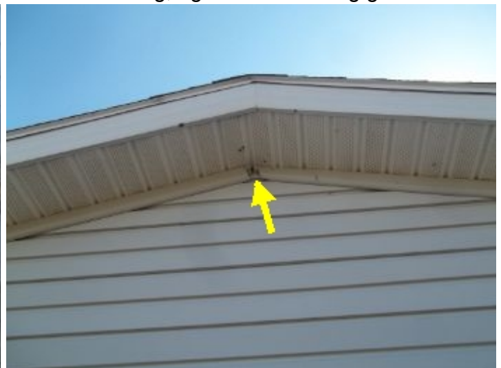
Gap in the top finish trim
