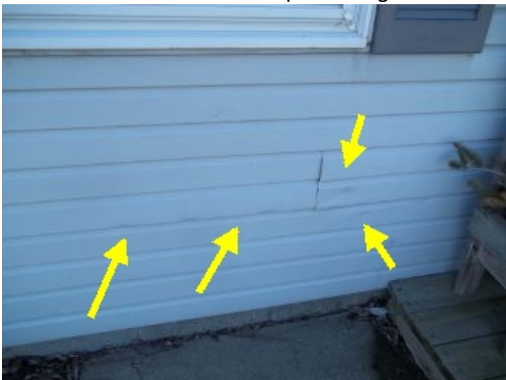
Damaged siding on the front of the house
