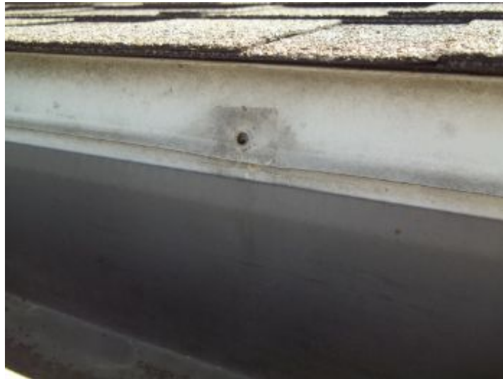
holes need sealed
