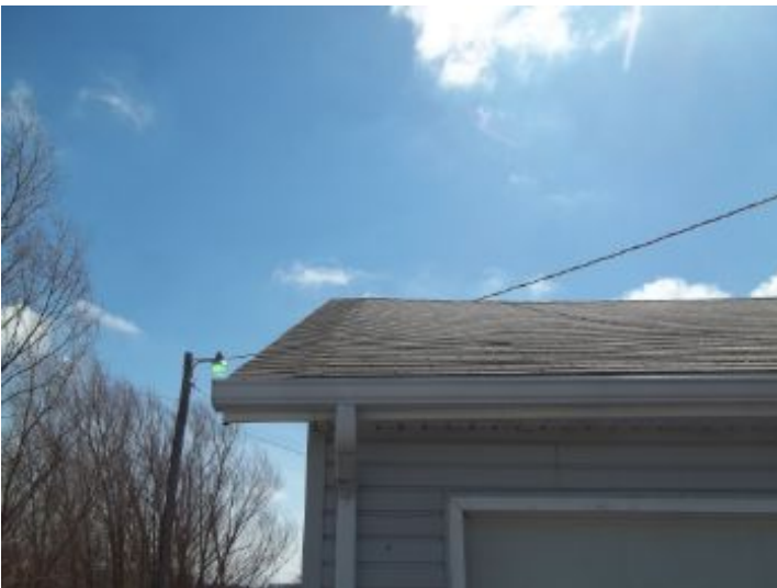
East side gable overhang sagging
