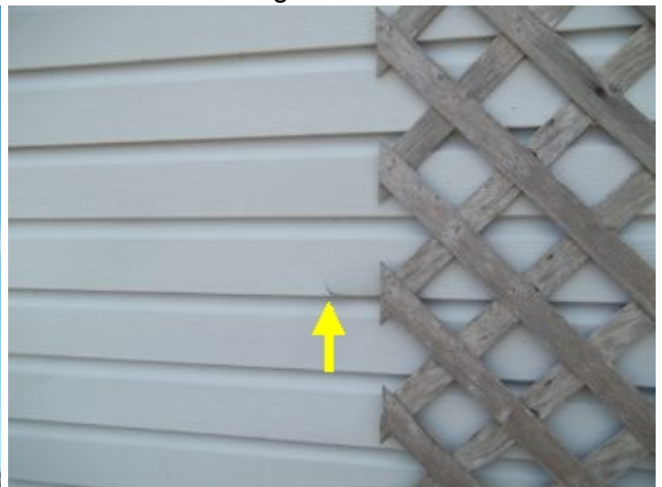
Crack in siding
