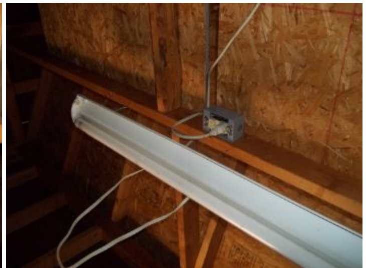
Cover plate missing
