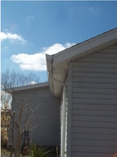
Roof and wall bowed out from roof sagging
