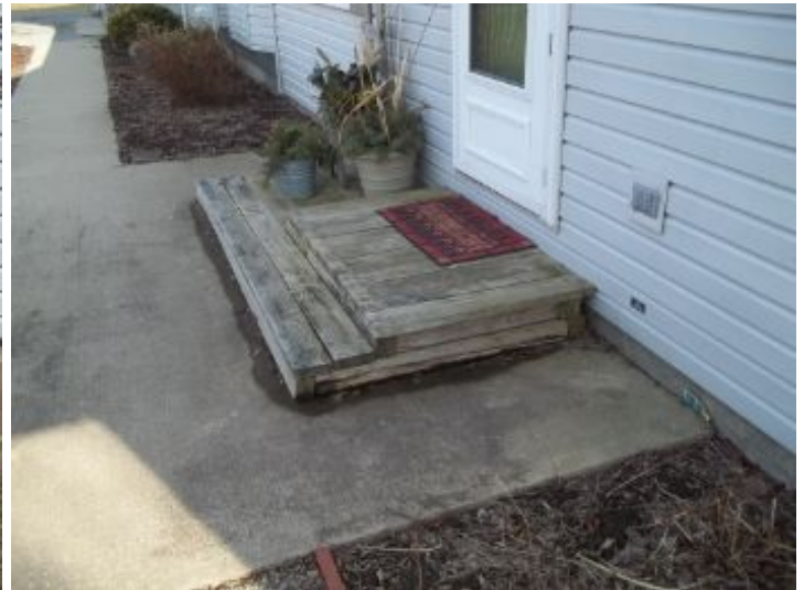
Front step is starting to rot at the bottom, where it is in contact with the concrete
