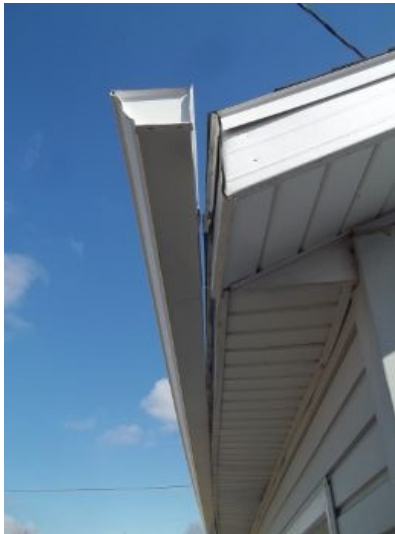
Gutter loose on front of garage and front wall and roof bowed out
