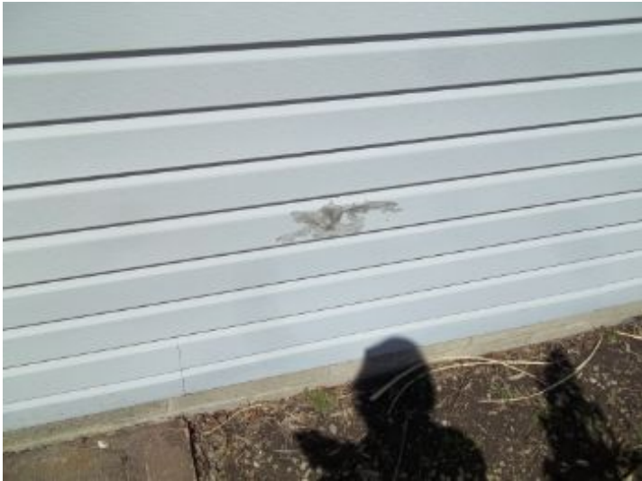
Caulk used to repair siding
