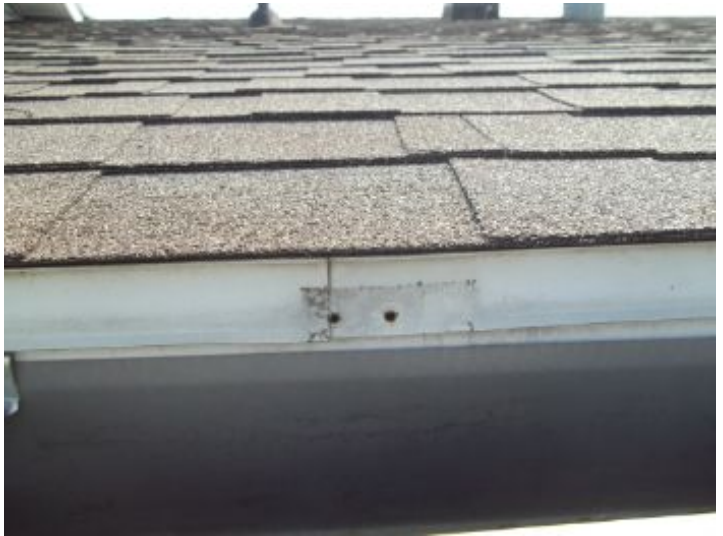
Holes need sealed where the old gutters were removed
