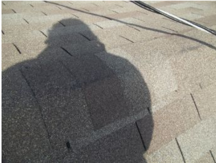
Ridge cap being damaged by the utility overhead service drop cable
