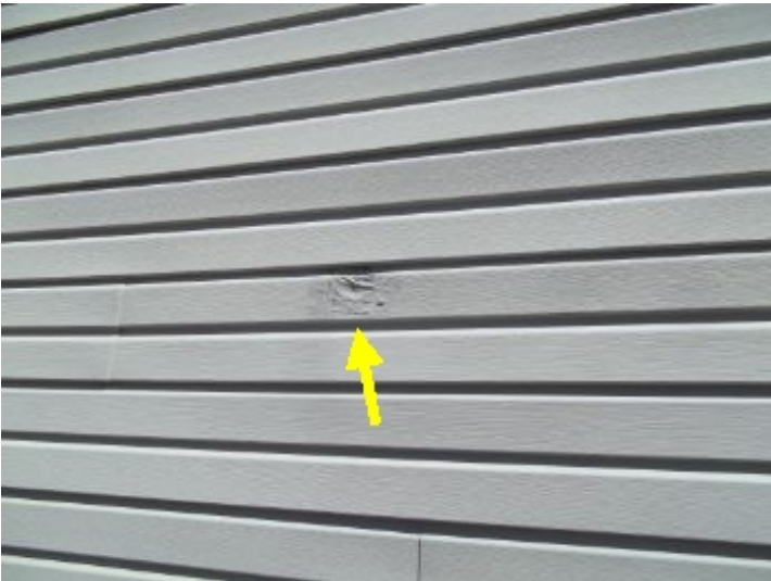
Poor repair/patch
