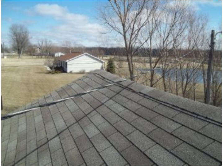
Improper clearance on utility service drop
