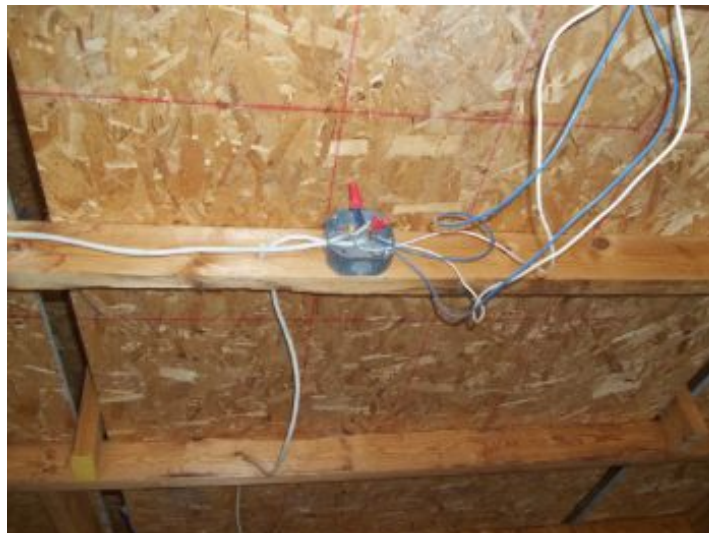
Cover plate missing, cable connectors missing
