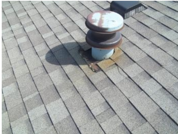
Furnace vent stack needs cleaned and painted
