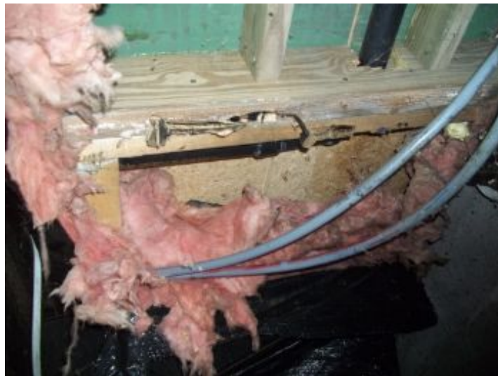
Bottom board damaged insulation missing
