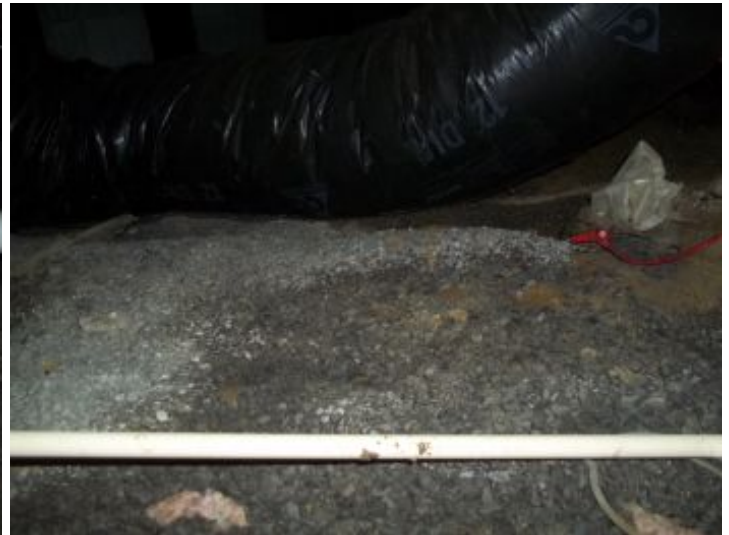
Crossover duct is lying on the ground
