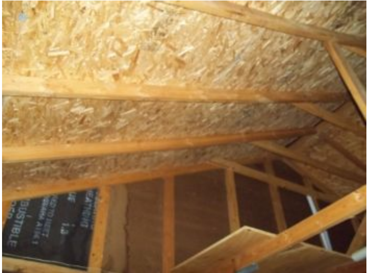
Dangerous roof framing, not to any building standards
