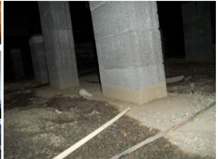
Evidence of prior water intrusion was found in one or more sections of the crawl space.
