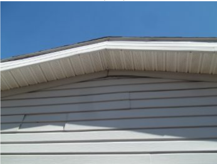
Loose siding and top piece of siding missing
