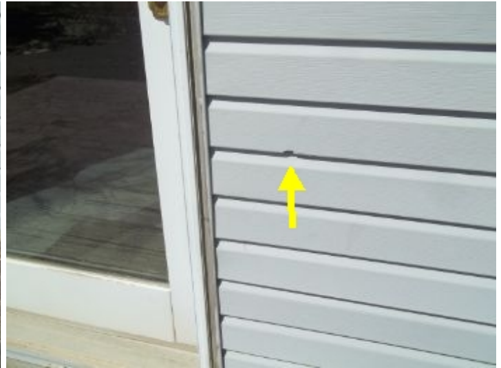
Hole in siding, right side of sliding glass door
