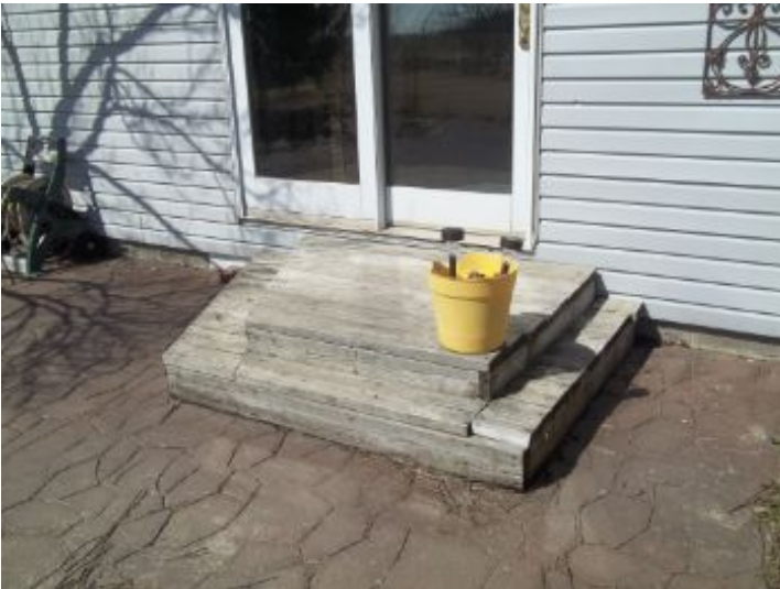
Wood steps to sliding glass door needs cleaned and sealed
