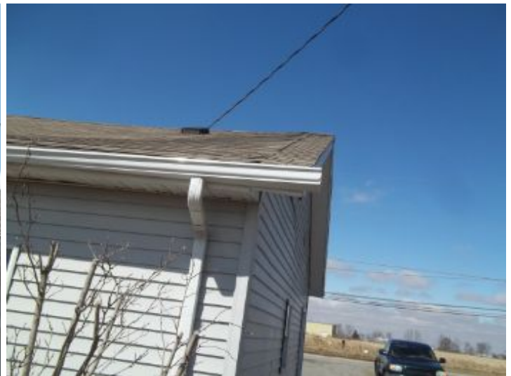
Garage rafters sagging
