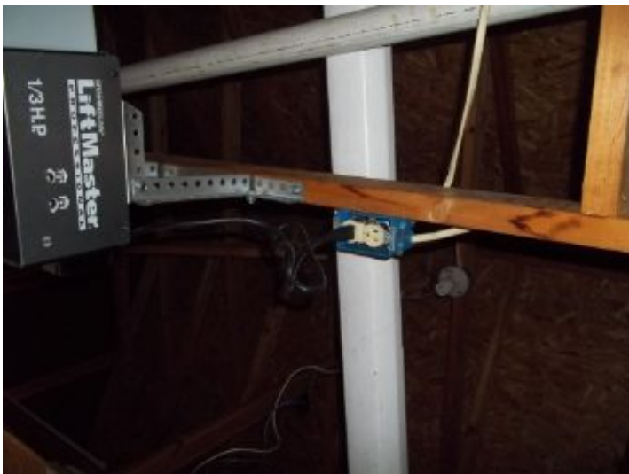
cover plate missing
