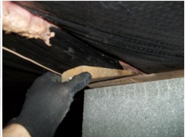
Suggest checking all the shims on the piers and tightening them as needed
