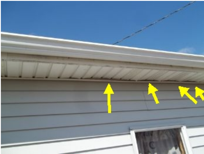
Soffit loose on the back of the garage
