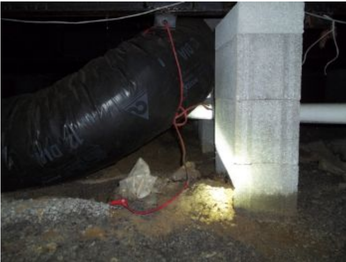
Duct not properly supported
