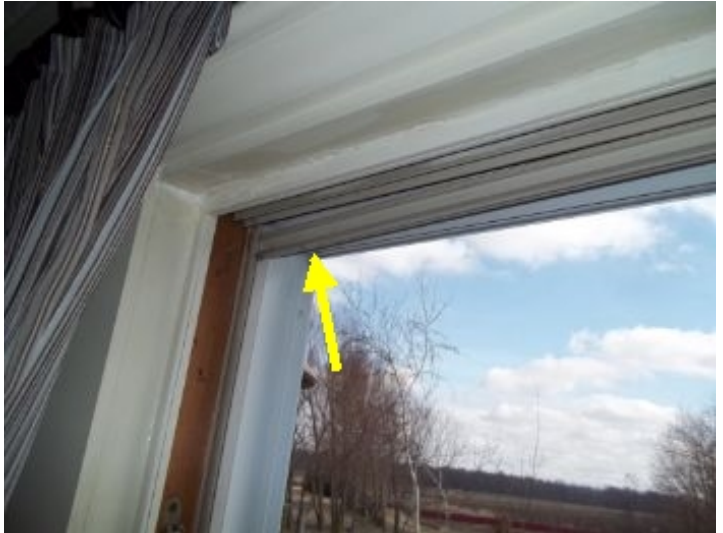
Loose seal trim on the sliding glass door
