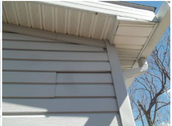
Loose siding west side of house
